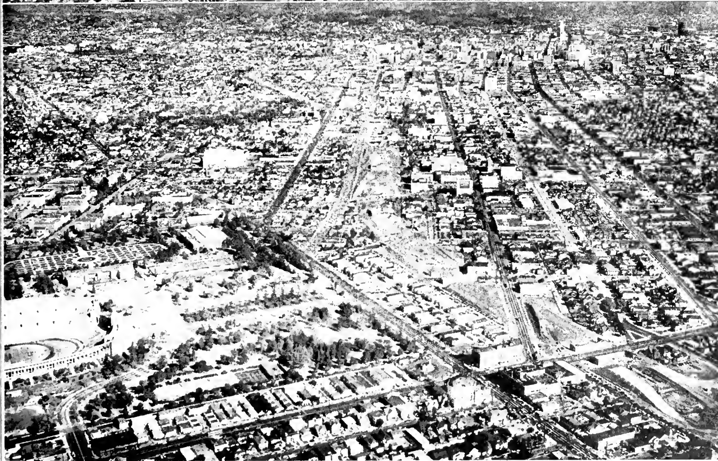
UPPER—Looking northerly along right of way that has been cleared of buildings for future construction on the Harbor Freeway. The traffic arterial on left is Figueroa St., next is Broadway and beyond is Main St. The east and west cross street, portion of which is shown foreground right, is Florence Ave. LOWER—Looking northerly along section of Harbor Freeway under construction between 23d St. shown just above center and 42d St. at right beyond limits of picture. The Los Angeles Memorial Coliseum is shown foreground left and Los Angeles downtown business district and Civic Center buildings, background right.
